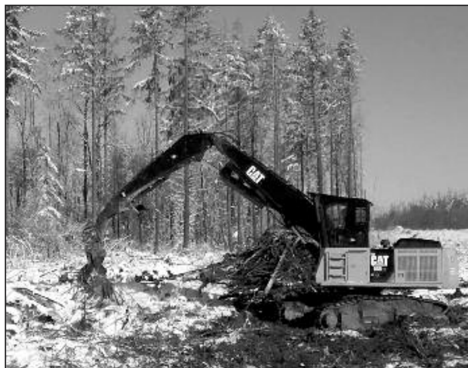
PILING BRUSH Holbrook's CAT 568 cleaning up.
