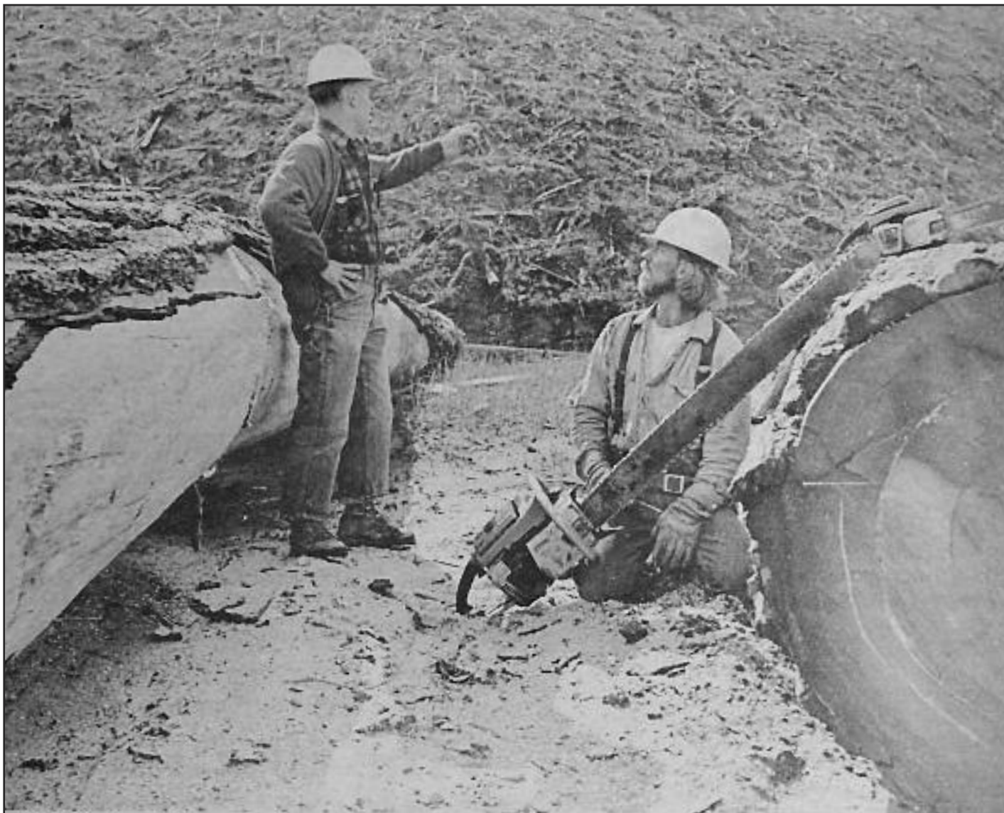
Dennis Hadaller (L), owner of Dennis Hadaller Logging talks with his hook tender, Jack Chambers of Centralia, WA. Jack was sharpening his chain prior to having another try at a log he was trying to cut in two. Jack kept hitting ash deposits which dulled his chain.
